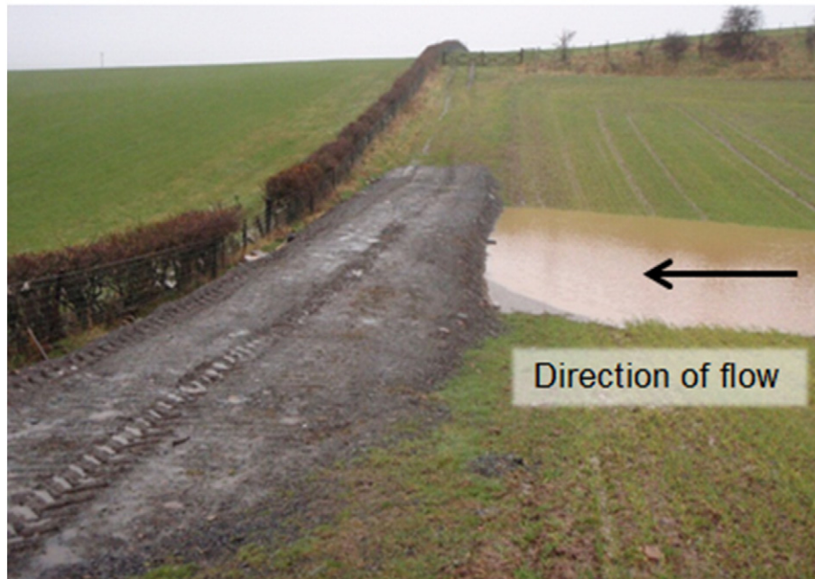
Fig. 5. A field bund RAF storing water during a storm.
