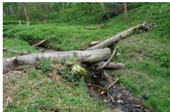
Figure 22 – Timbers placed in cross formation
