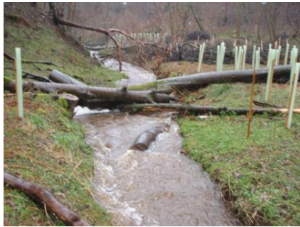
Figure 26 – Large Woody Debris Dam
