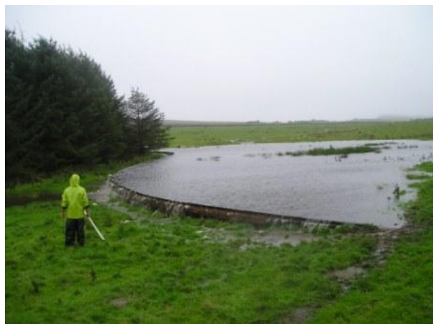
Figure 4 – Offline Storage Pond constructed of leaky timber barrier so as to release flow slowly back to the river
