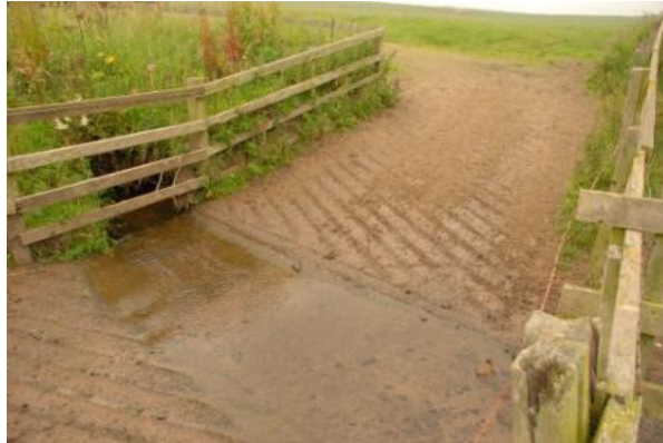
Figure 34 – Dedicated crossing and watering point for livestock
