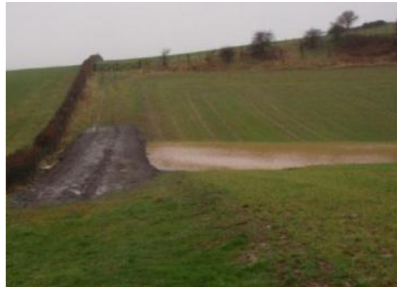
Figure 19 – Field bund, acting as a raised access track, storing overland flow during heavy rain
