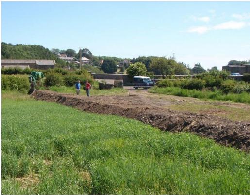
Figure 18 – Bund being constructed across primary flow pathway
