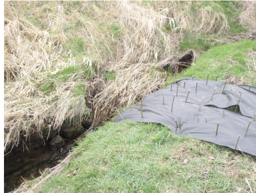
Figure 32 – Willow Hurdles to slow and attenuate flood flow
