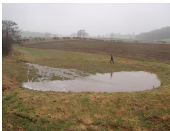
Figure 8 – Offline pond starting to fill during heavy rain
