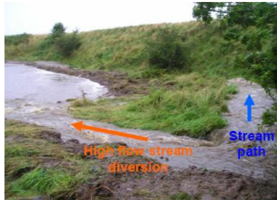
Figure 3 – Spill point created by lowering river bank on the outside of a bend
