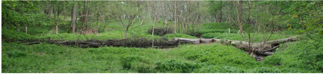
Figure 28 – Large Woody Debris dam plus pinned brush barrier on flood plain
