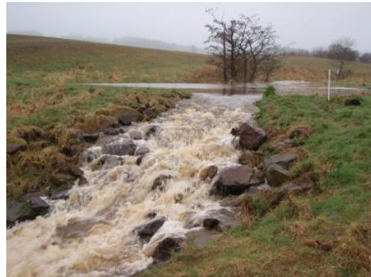
Figure 11 – Rock Armoured spillway on an online pond during flood conditions
