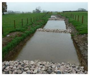
The ditch of the future. How to hold water during storms to maximise flood retention, to recharge the aquifer and lower diffuse pollution. Taken from the Defra Demonstration Test catchment Programme (Barber 2014).
