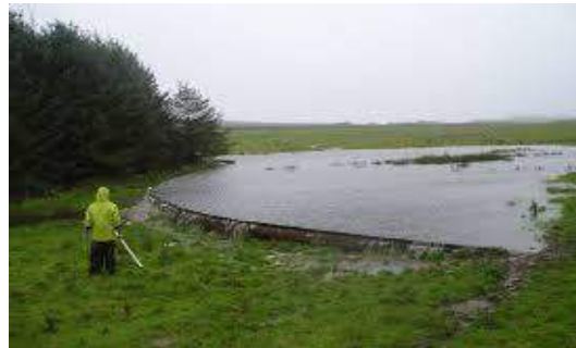
Medium sized JOHAD (check dam) Rajasthan, India, recharges dry underground aquifers
