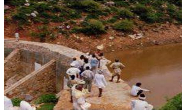
Medium sized JOHAD (check dam) Rajasthan, India, recharges dry underground aquifers
