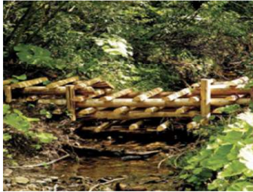
Slovakia – wooden mesh intervention slows flood waters upstream
