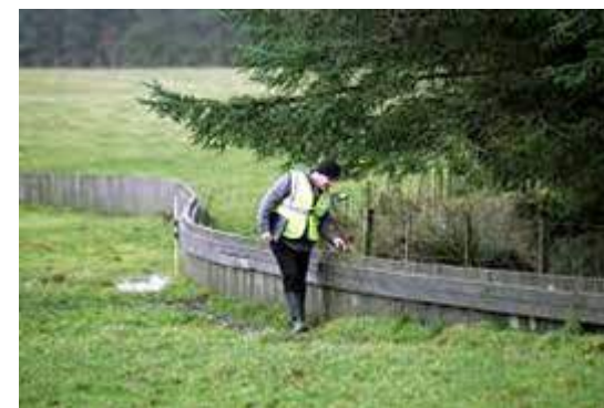
An iconic 'bund' to stop flooding, Belford, UK
