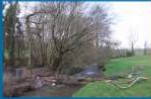
Woody debris installed in Belford Burn
