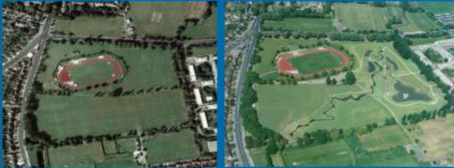
River Quaggy at Sutcliffe Park, South London, before and after flood alleviation work
